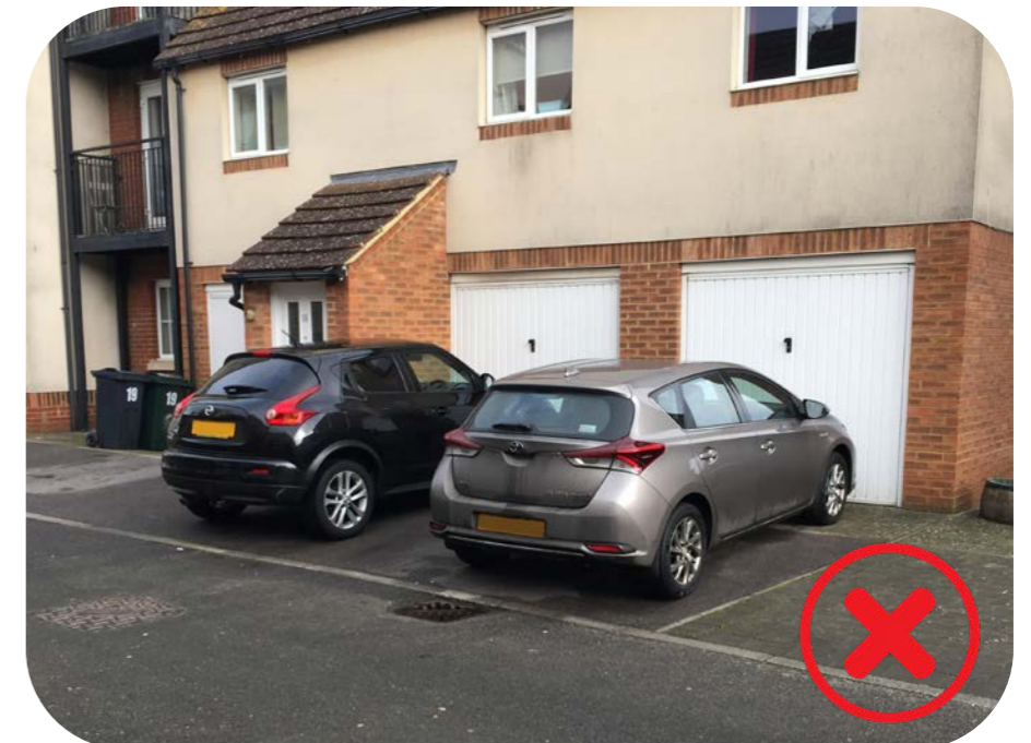
Driveway Insufficient to allow for Access to Garage resulting in Carriageway Overhang, Repton Park, Ashford
