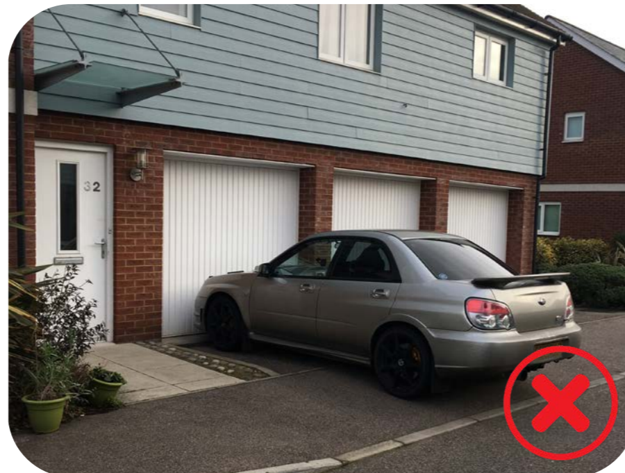
Insufficient Garage Set Back can Result in Vehicle Overhang, Springhead Parkway, Gravesend
