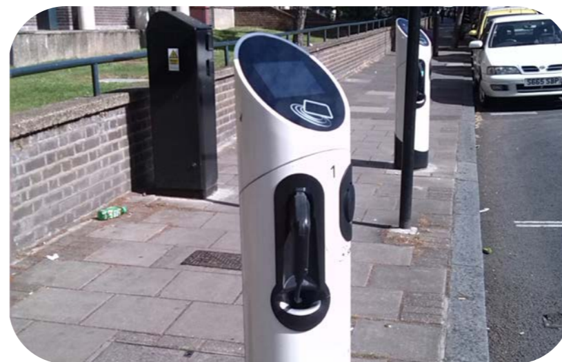
On-Street EV Charger
